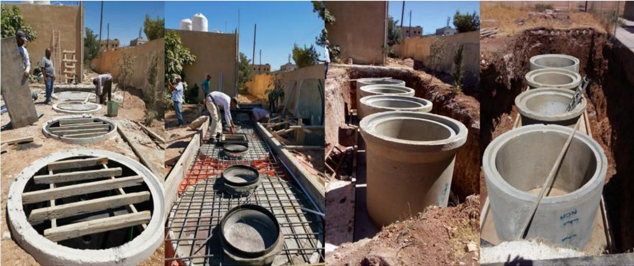
Figure 1: Decentralized wastewater treatment plant using the Modified Septic Tank technology installation in Rehab Schools.
