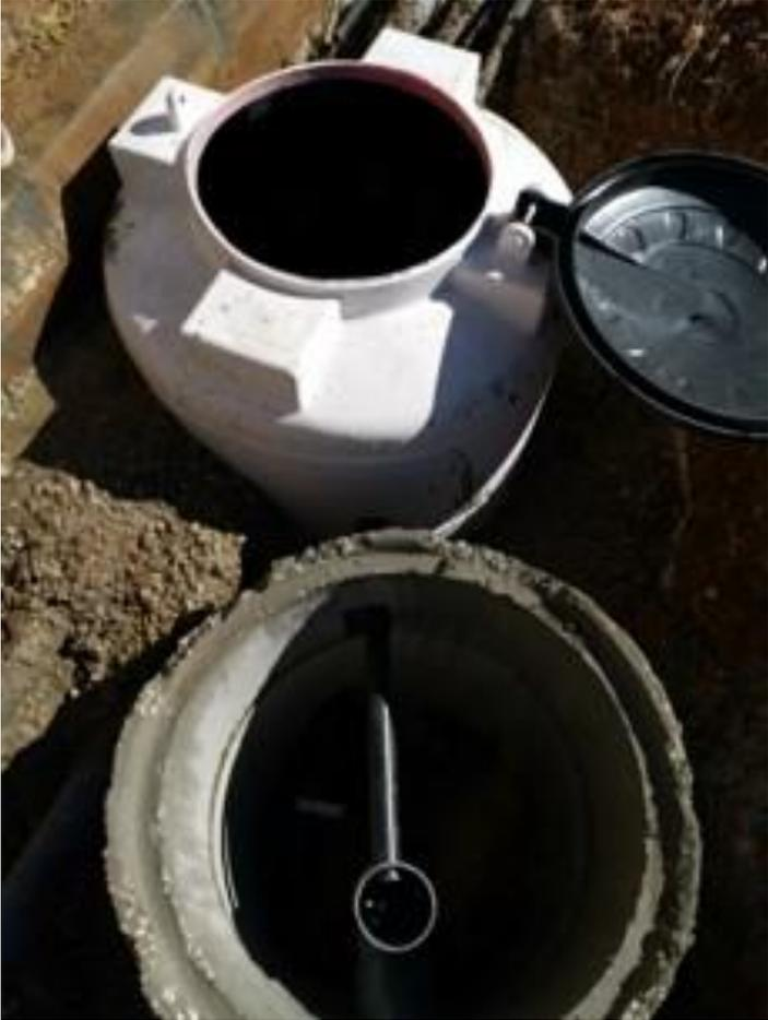
Figure 2: Gray water treatment and reuse installation in Rehab Schools.
