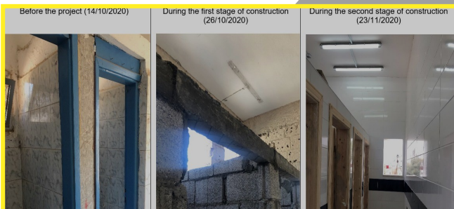
The toilets renovation at Al-Khansa'a Elementary Mixed School
