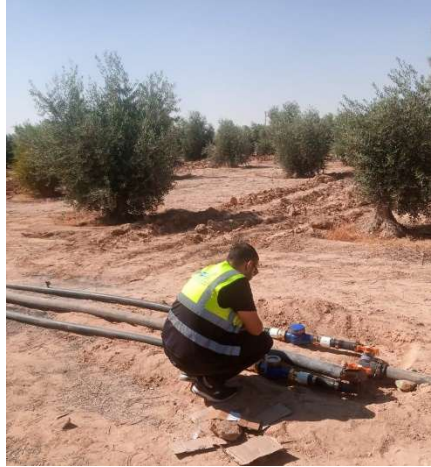
Picture 2: MIRRA trainee installing sustainable irrigation systems to conserve water and enhance soil health in Azraq farms
