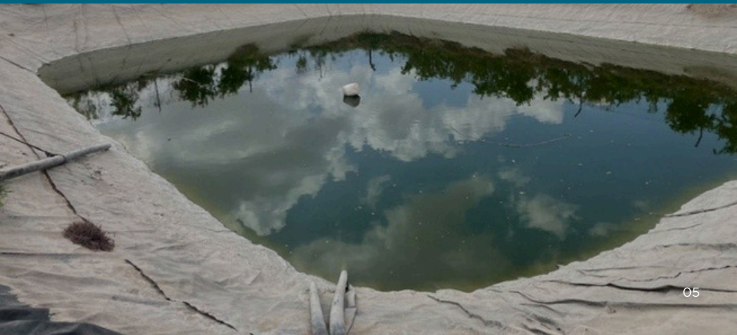
Picture 2: A plastic-lined pond commonly used in the Jordan Valley to store water.
