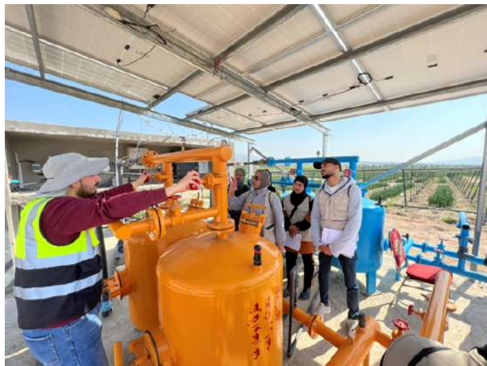
MIRRA's Irrigation Engineer Khalil Bany Mustafa (left) explains the process of sand filter back flushing for a group of young professionals from the Jordan Valley
