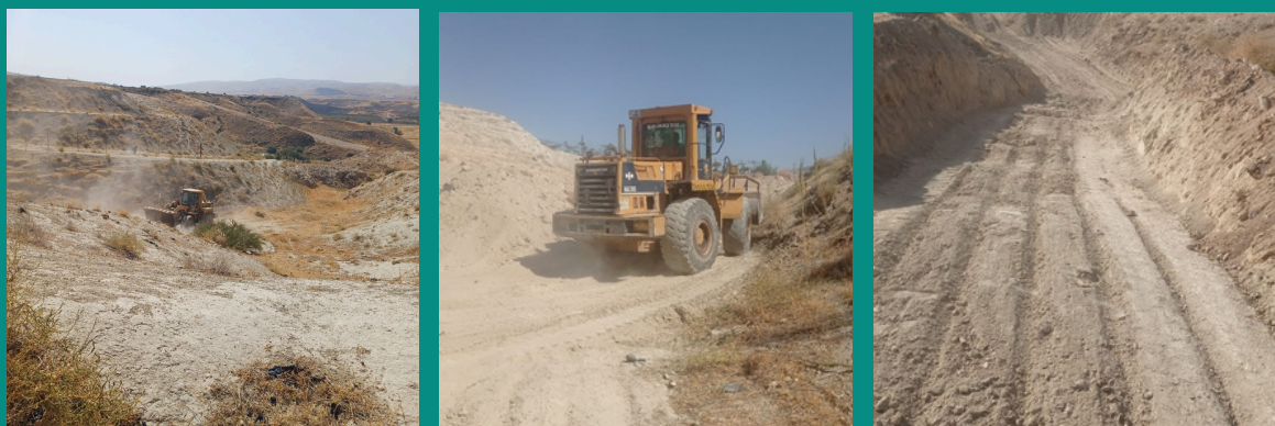
Picture 3: Stages of preparing a rainwater harvesting pond, including cleaning, reshaping the site and preparing it.
